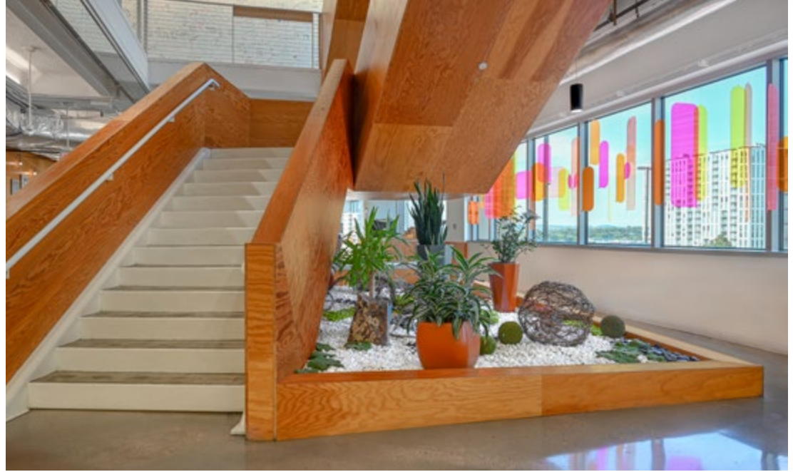
Staircase connecting Floors 9 thru 12
